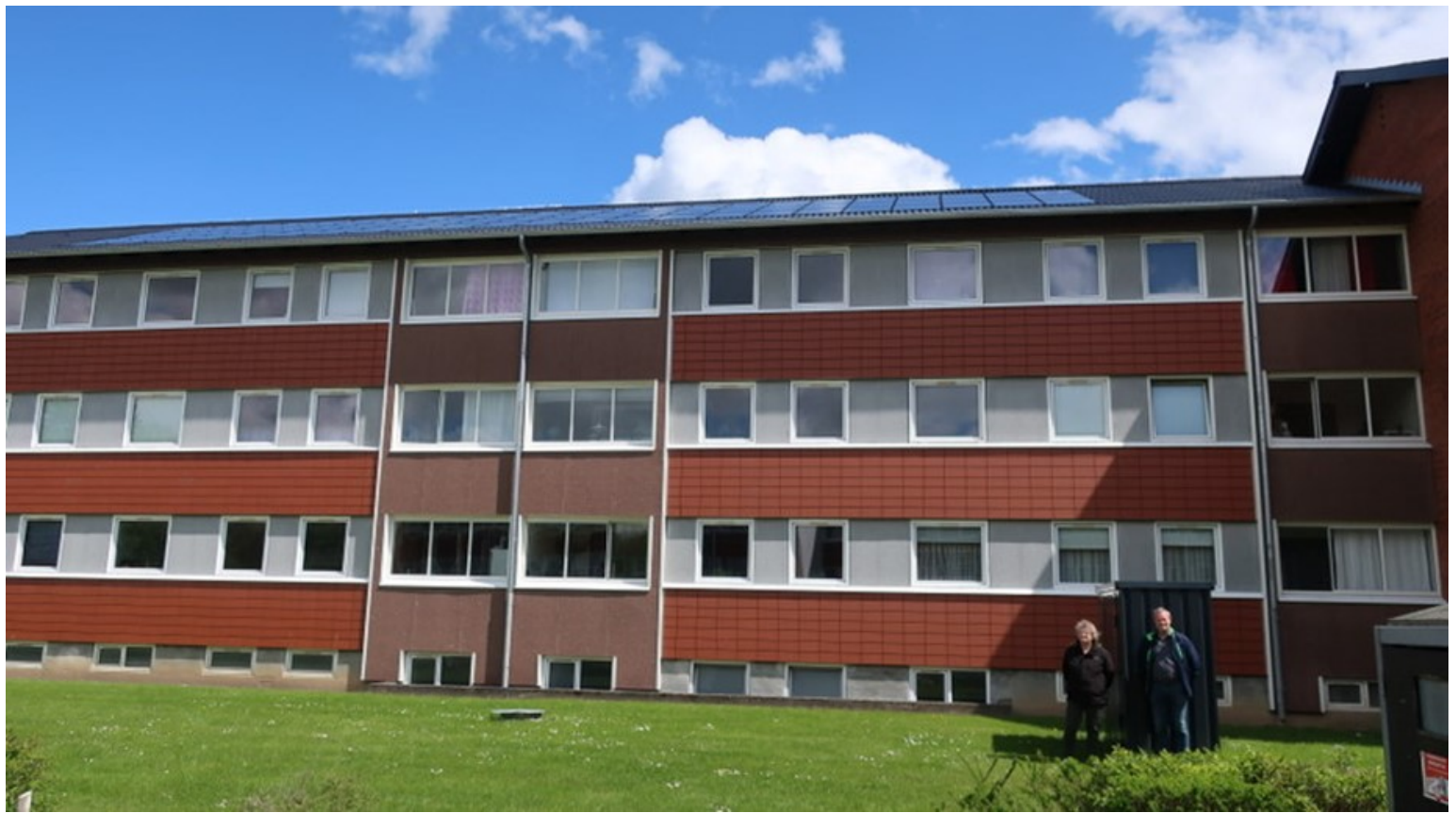
Søbo's department 12 with roof-integrated solar cells and battery cabinet
